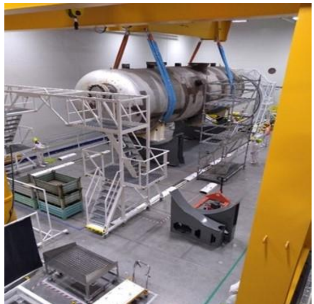
Fig. 24 and 25: Transport of steam generator PG 11 to SO 490 V-1
