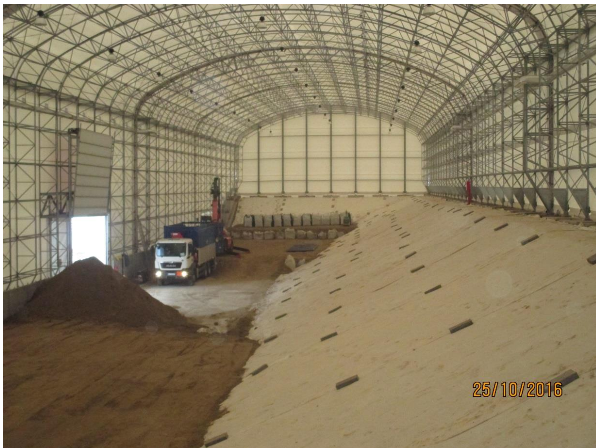
Fig. 22: Disposal of VLLW in the first stage of VLLW repository with a disposal capacity of 20 000 m 3 for RAW from the decommissioning of NPP A-1
