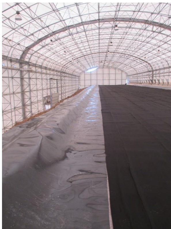
Fig. 22: Disposal of VLLW in the first stage of VLLW repository with a disposal capacity of 20 000 m 3 for RAW from the decommissioning of NPP A-1
