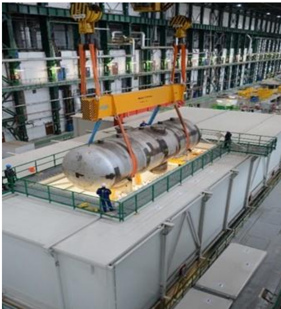
Fig. 24 and 25: Transport of steam generator PG 11 to SO 490 V-1
