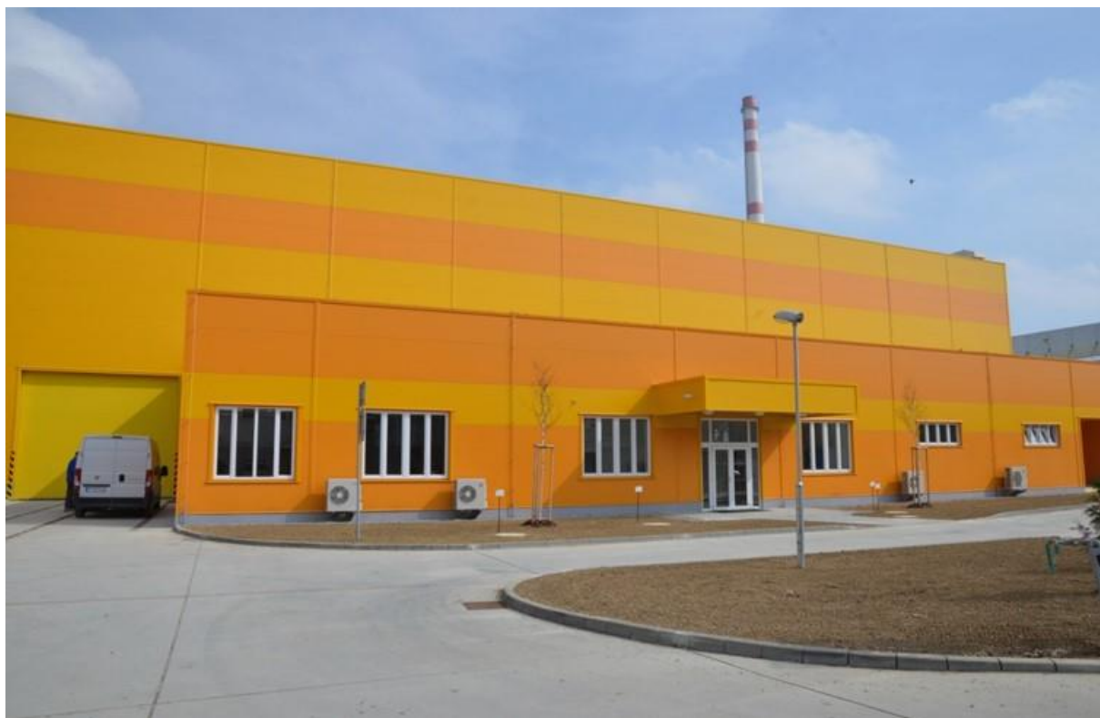
Fig. 5 Integral Storage Facility for RAW
