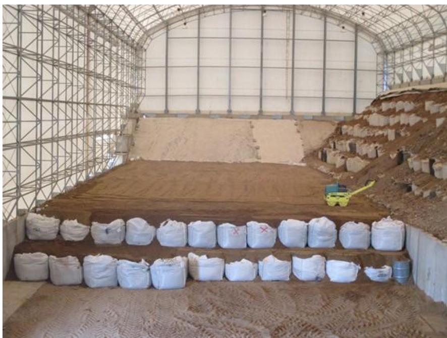
Fig. 10 Disposal of VLLW in the first stage of VLLW repository
