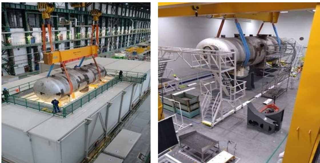
Fig. 12 Transporting steam generator PG 11 to SO 490 V1
