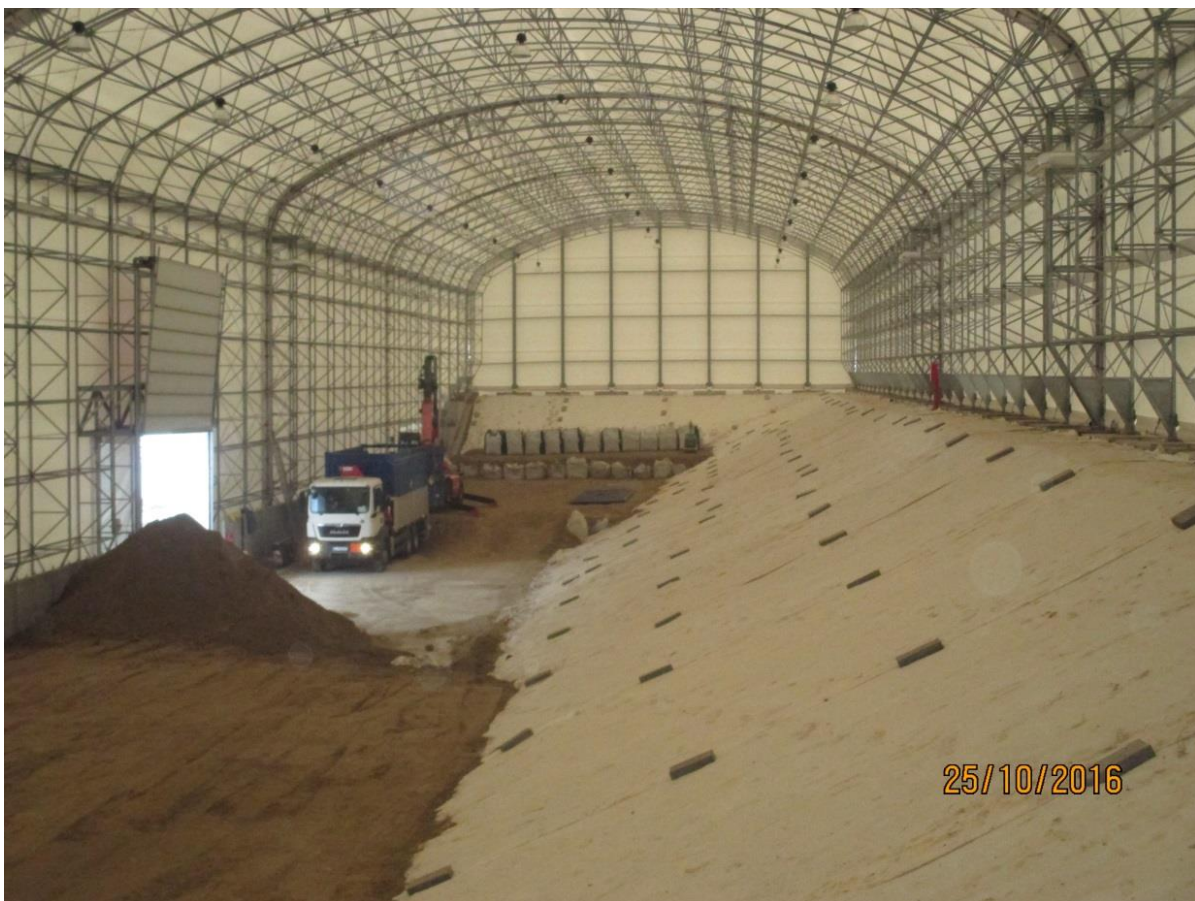
Fig. Disposal of VLLW in the first stage of VLLW repository with a disposal capacity of 20 000 m 3 for RAW from the decommissioning of NPP A 1
