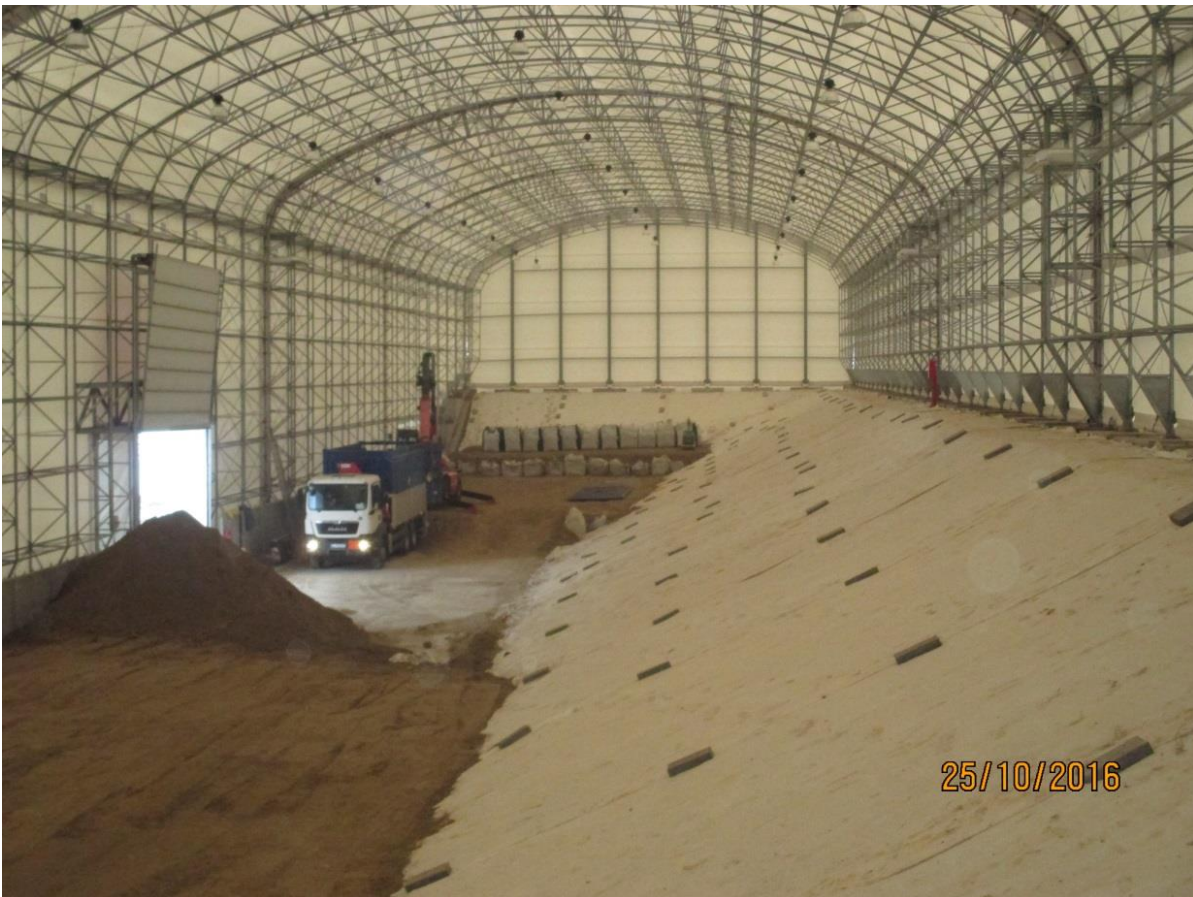
Fig. 20: Disposal of VLLW in the first stage of VLLW repository with a disposal capacity of 20 000 m 3 for RAW from the decommissioning of NPP A-1
