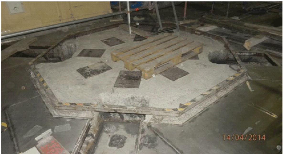
Fig. Seismic upgrading of the stand for portable seals (EMO 3&4)
