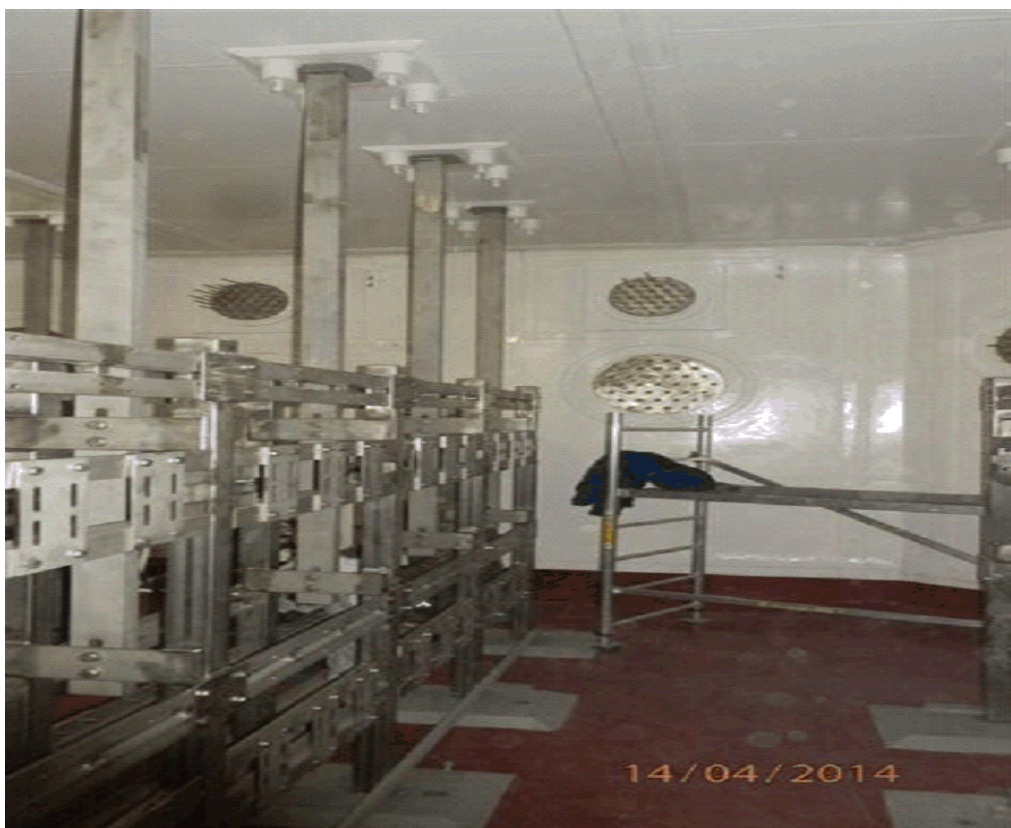
Fig. Seismic upgrading of the I&C (instrumentation & control systems) room in the main reactor building (EMO 3&4)
