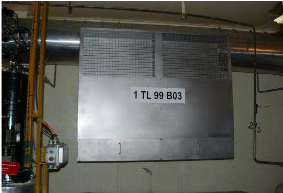
Fig. Installation of passive autocatalytic hydrogen recombiners
