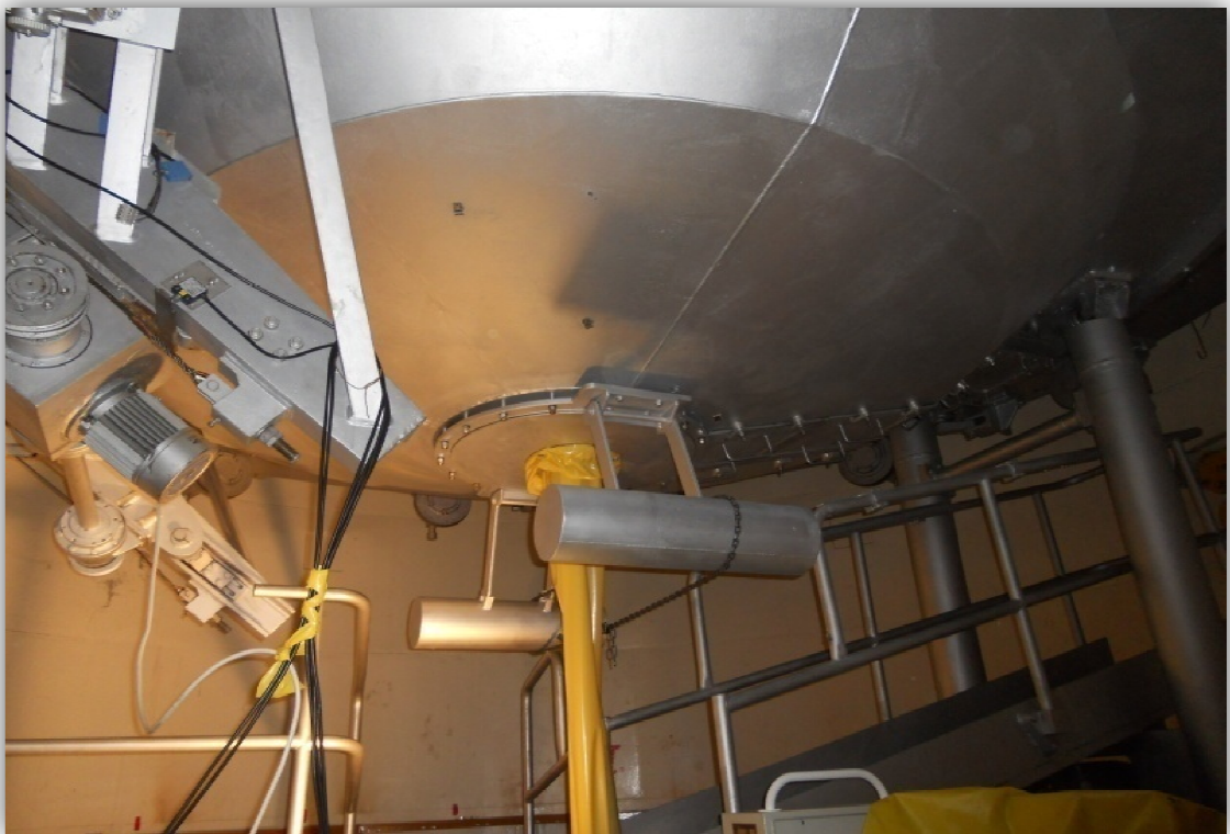
Fig. Bottom part of reactor shielding with floats for outside-zone cooling of RPV
