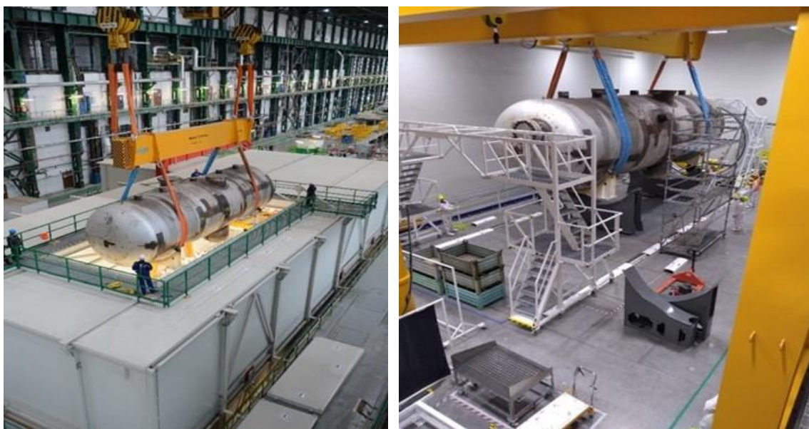
Fig. 13 Transporting steam generator PG 11 to SO 490 V1
