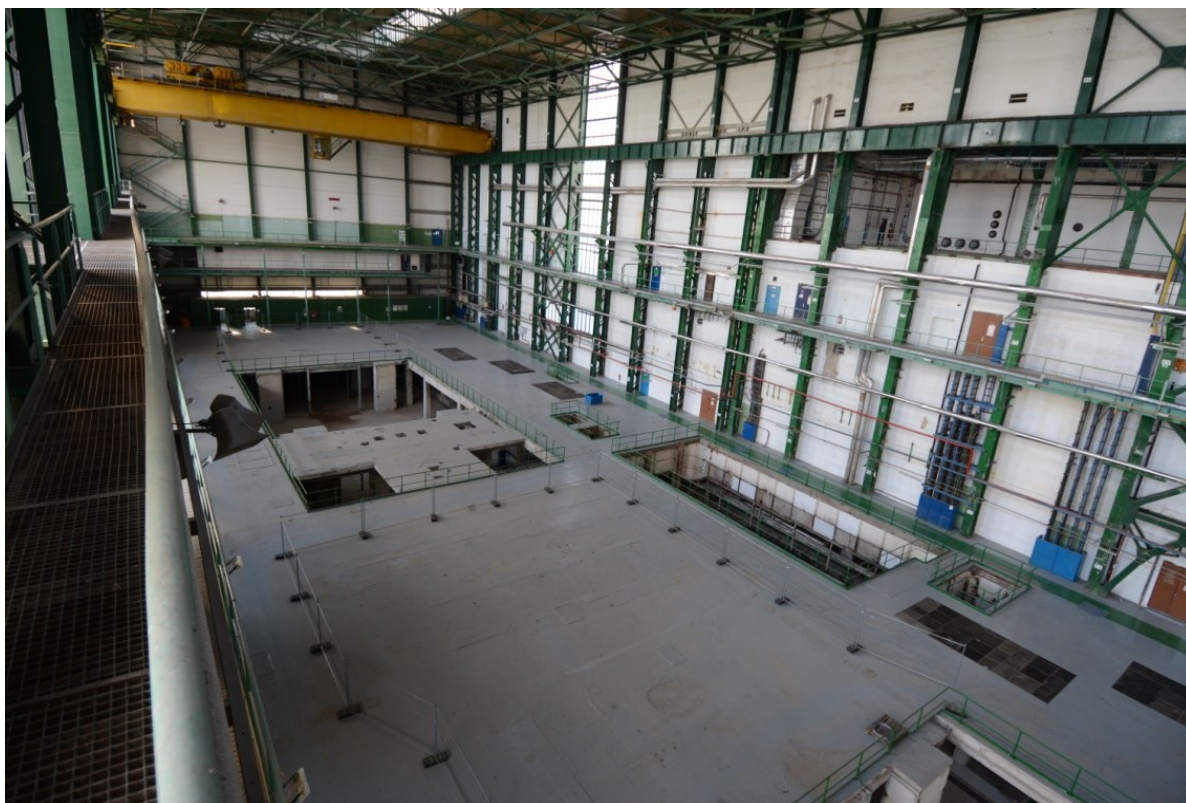
Fig. D.3.1 Machinery room after dismantling of the technological part
