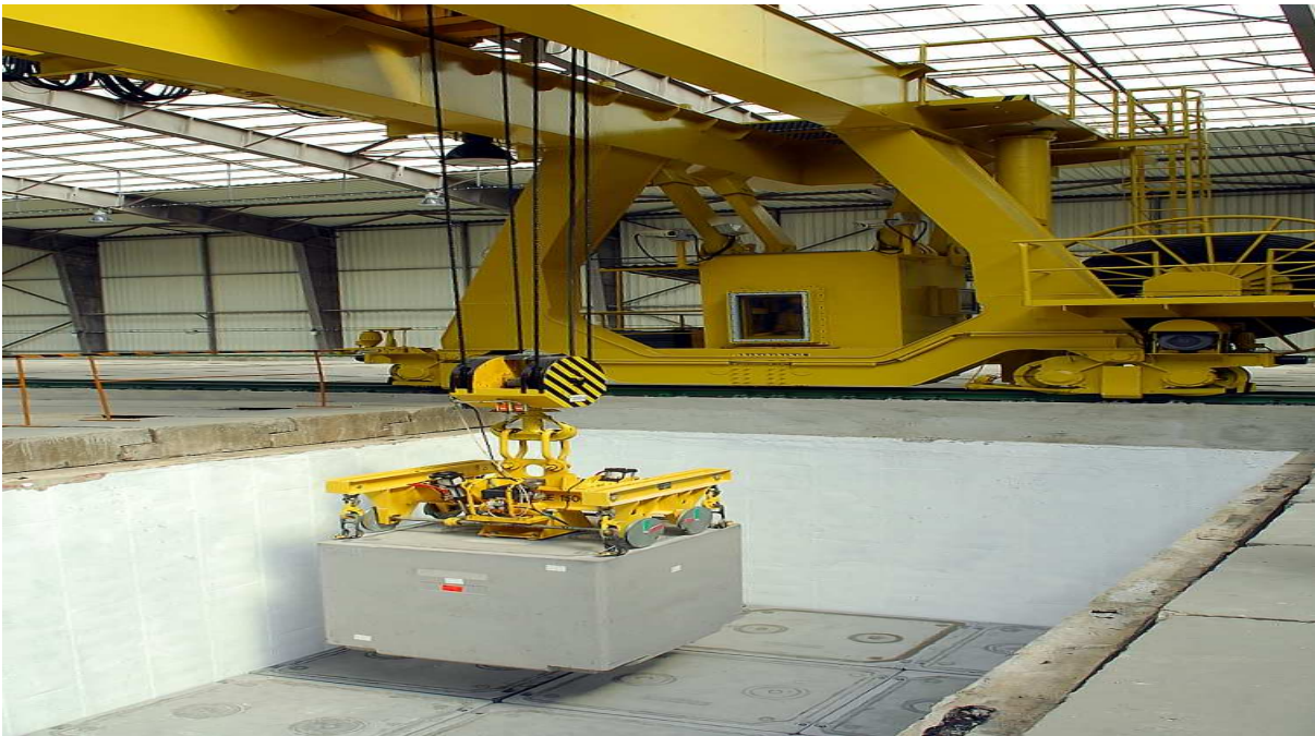
Fig. Disposal of VBK to disposal boxes of the repository in the first double row
